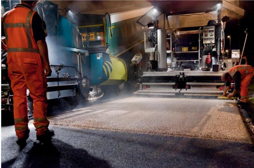
Figure 1: The first metres with clear binder (section C) on A35
