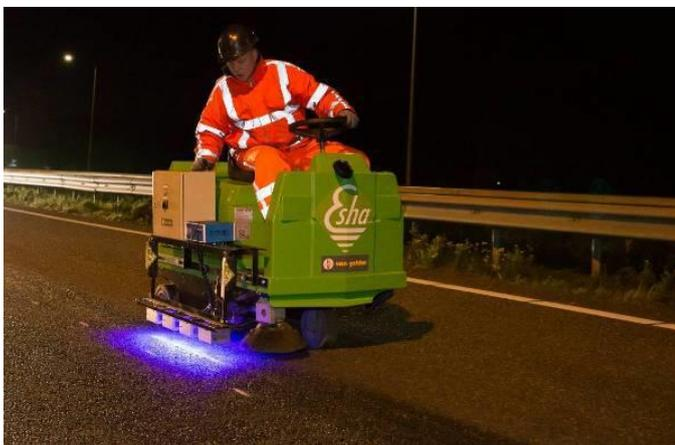
Fig. 7: One of the 5 innovative joint protectors that was successfully validated
