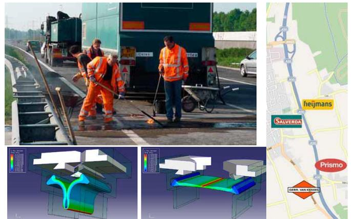
Fig. 6: Long lasting joints project, FEM simulations in smallest (bottom left) and largest (bottom centre) opening, locations in the highway A50 where four products were field tested (right) and construction photo (top)
