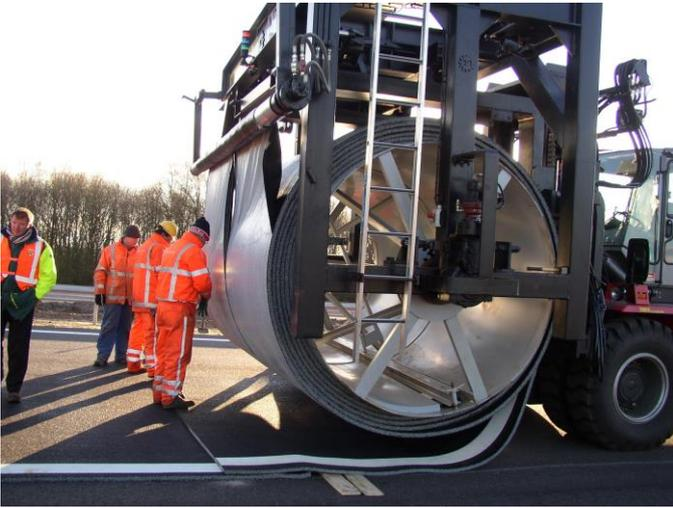
Fig. 4: Rolled up asphalt concrete
