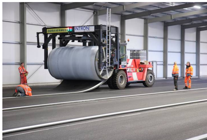
Figure 3: After production the asphaltmat is rolled on the reel.
