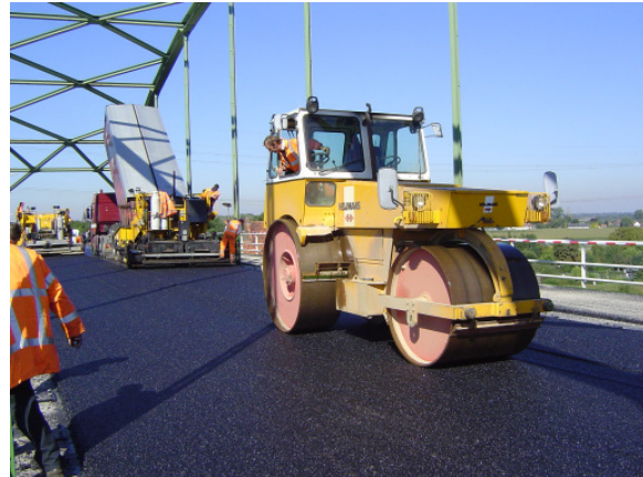
Figure 7: Compacting like normal asphalt
