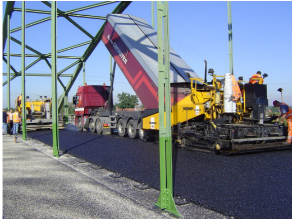
Figure 6: Paving the asphalt at the membrane
