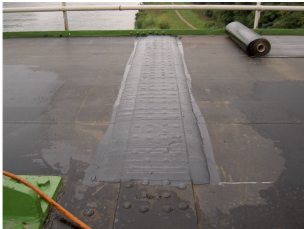
Figure 4: Levelling the steel strips
