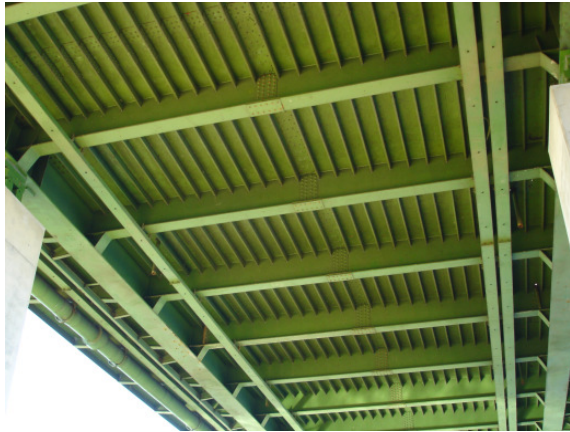
Figure 1: Orthotropic steel bridge deck
