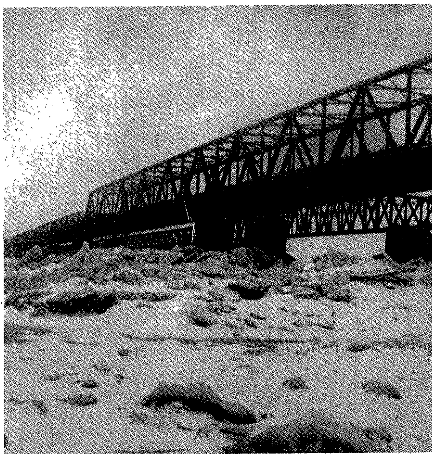
Fig. 5 Ice dam Zaltbommel 1942, downstream the bridges. The height of the ice above the water level is partially 4 m and more.
