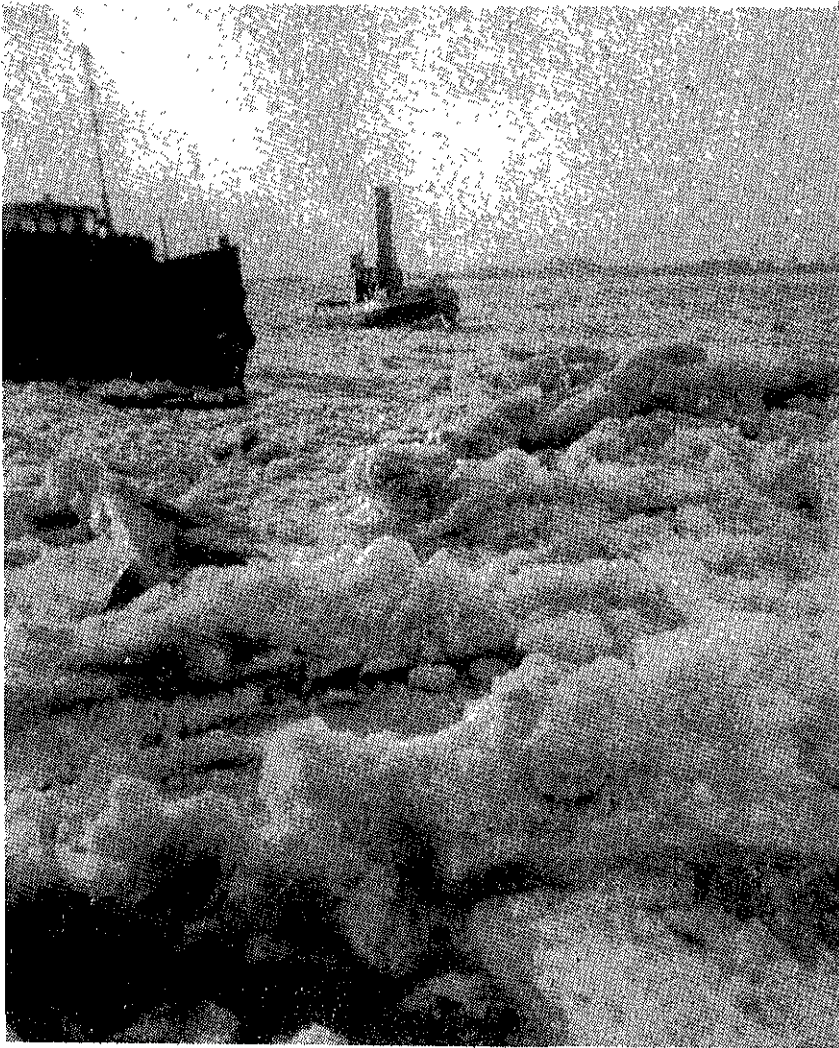
Ice breakers working on the Waal, 1954.
