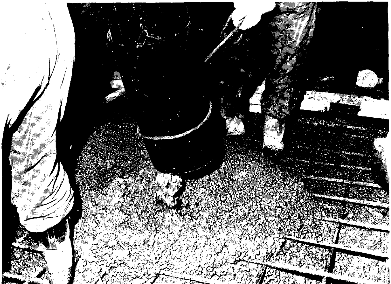
Figure 5. Placing the lightweight concrete
