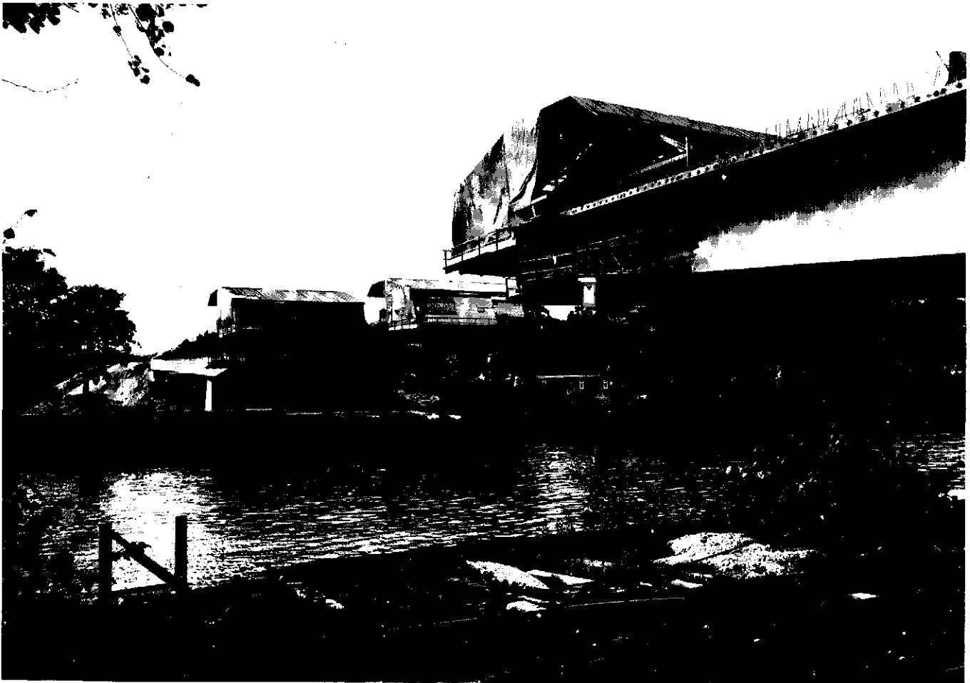
Figure 4. Cantilever construction of first bridge (October 1971)
