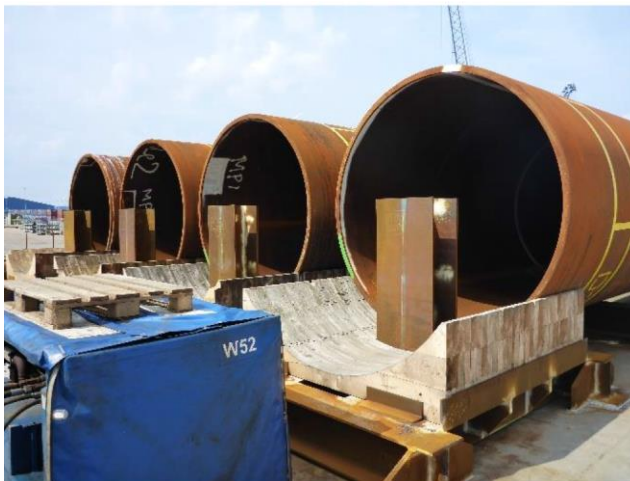
Figure 15: Example of upending frame with hard wood (to be considered lost after use)
