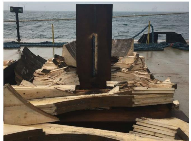
Figure 15: Example of upending frame with hard wood (to be considered lost after use)
